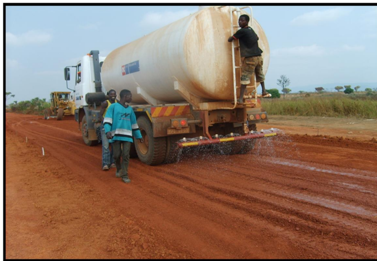
Figure 7 - Spray-on technique of EL-SSS with tanker
